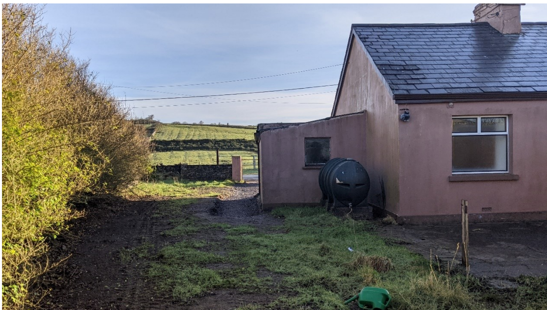
Plate 4-8 Part of the western elevation of the house.
